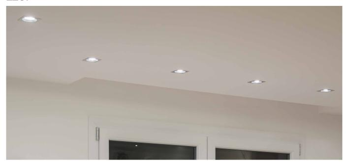
Polished, decorated aluminium recessed square light with powerful LEDs suitable for decorative lighting of residential and retail environments. Choice of secondary recessed optics. Can be flush fitted indoors. Flush-mounted with springs.
